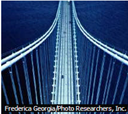
Frederica Georgia/Photo Researchers, Inc. Verrazano-Narrows Bridge
