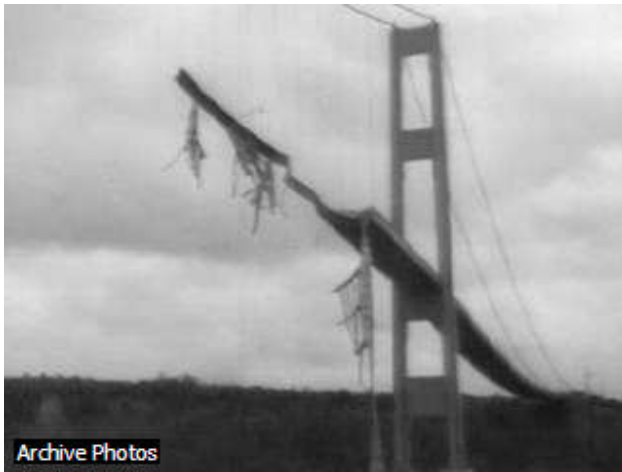
Archive Photos Collapse of the Tacoma Narrows Bridge
